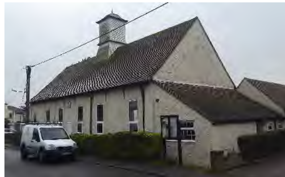
Figure 27 The Village Hall Manor Road
