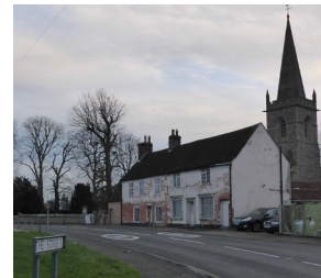
Figure 16 Grade II Listed 1 The Street (Church Cottage)
