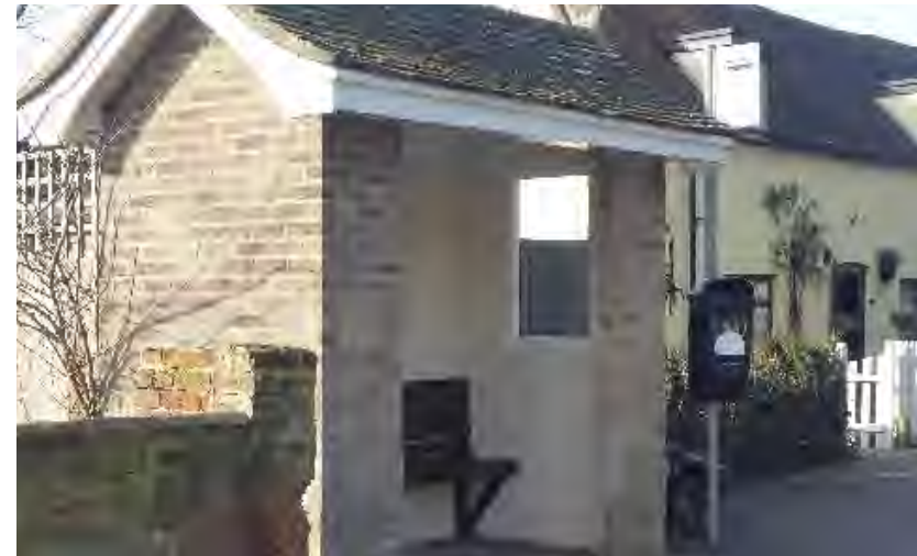
Figure 52 The bus shelter on Rectory Road
