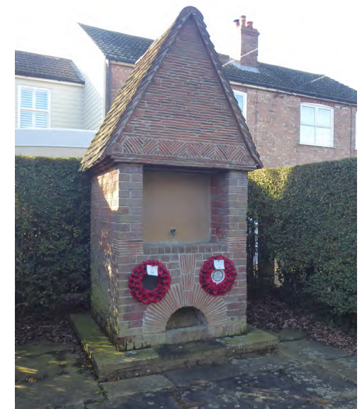
Figure 5 The War Memorial Drinking Fountain on Rectory Road
