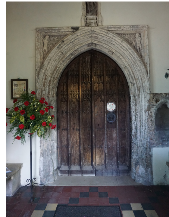
Figure 8 St Mary's Church door
